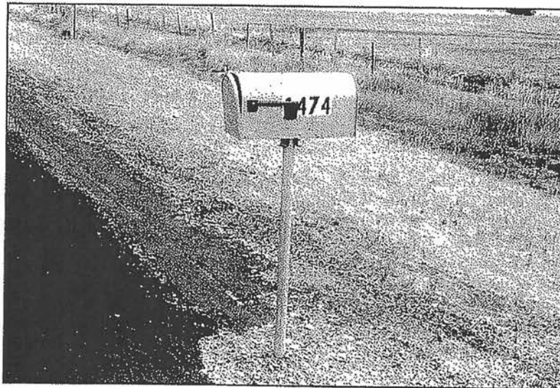
Figure 1B. Mailbox with Steel Post Support
