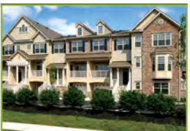
Heritage Pointe Chalfont, Bucks County
