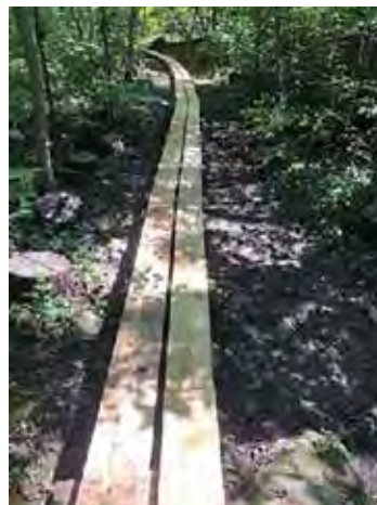
Part of the installed boardwalk.
