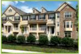
Heritage Pointe Chalfont, Bucks County
