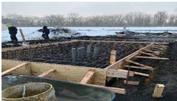
Framework for new generator pad
