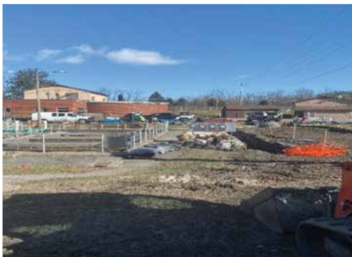
Concrete base for new aerobic air system
