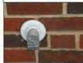
Sample Outside Vent for Indoor Gas Meter
