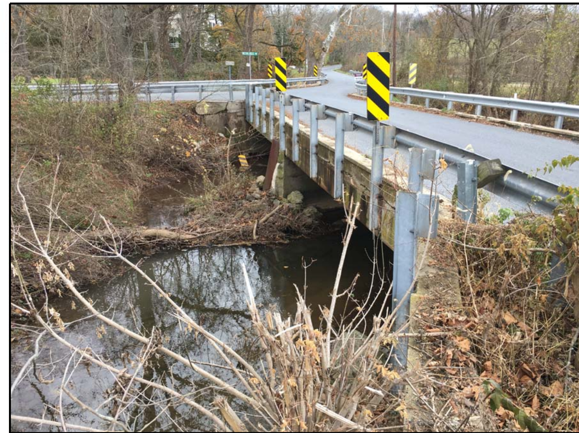
P-3: UPSTREAM BRIDGE ELEVATION LOOKING EAST
