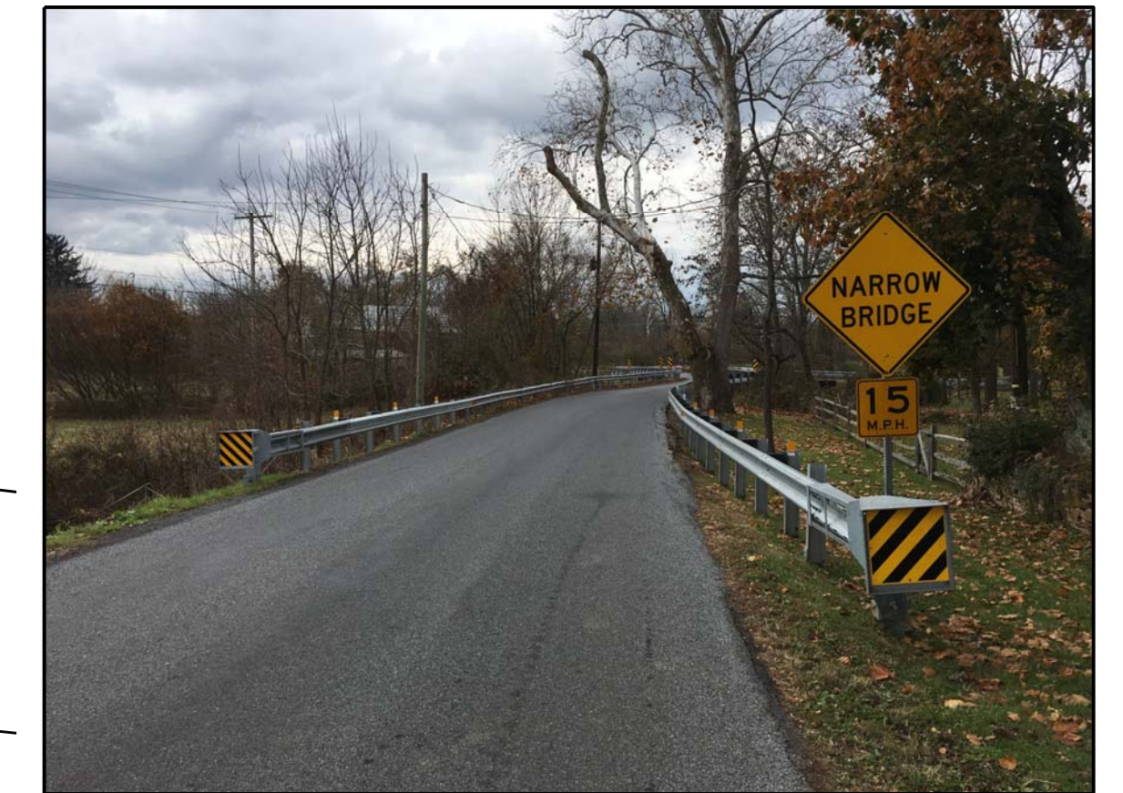
P-6: EAST APPROACH LOOKING WEST
