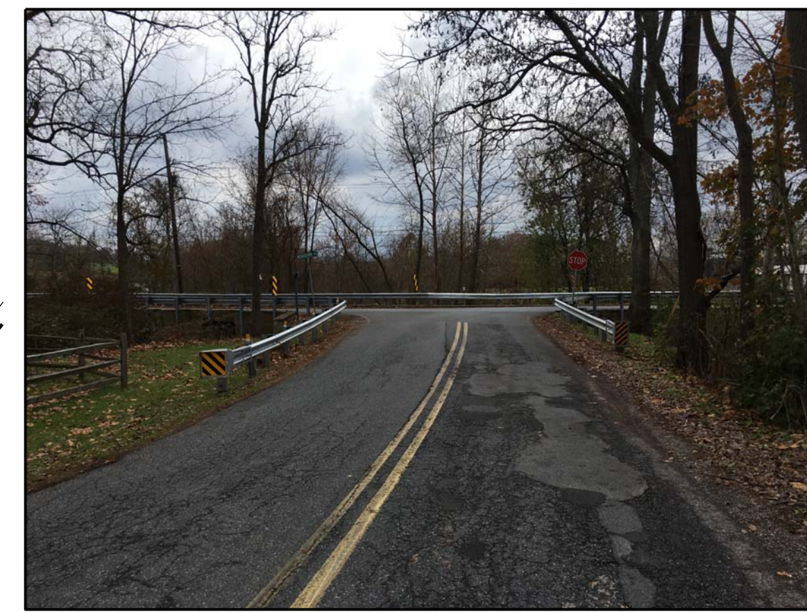
P-4: NORTH APPROACH LOOKING SOUTH AT THE INTERSECTION
